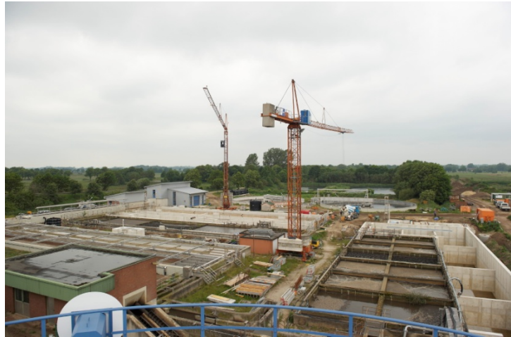
Overview of the treatment plant construction site
